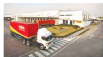
Makro Wang Noi Distribution Center, Ayutthaya province
